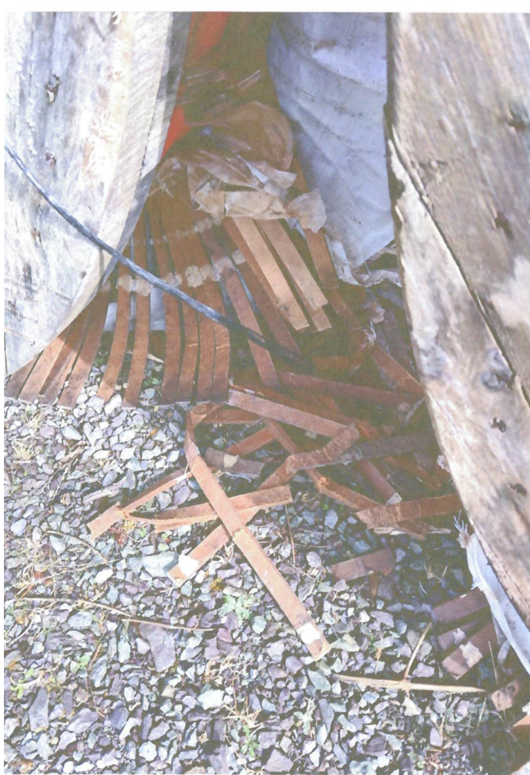
Photo 25 Camigdangan Meenbog cabling
